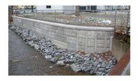
For an economical alternative to other eco wall systems, consider using environmentally friendly ecology blocks. Produced with high-strength, 5,000 psi concrete, each ecology block is cast with a groove in the bottom and a tongue on the top for a firm, secure fit and to prevent movement when stacked. With an attractive, paintable,
